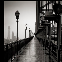
Michael Penn Ben Franklin Bridge
