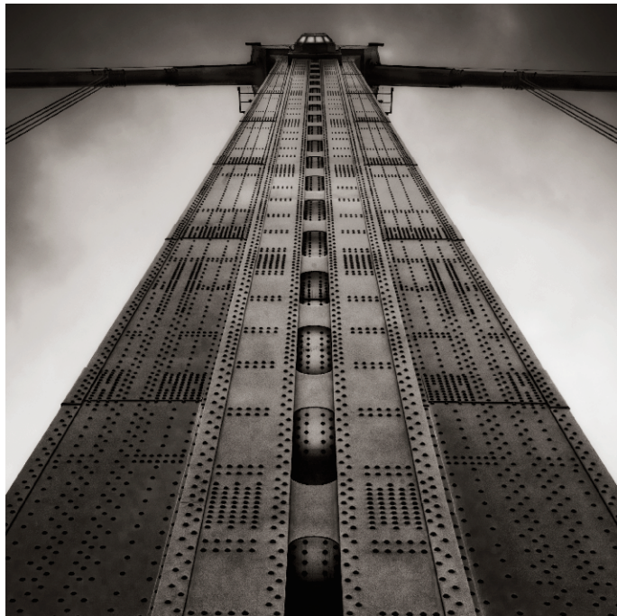
Cable Support, Night
